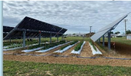
Tomato, eggplant & pepper under double wide single- axis tracker arrays
