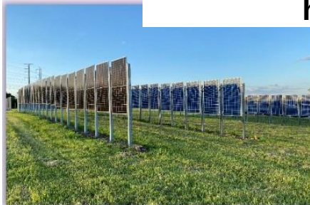
Vertical bifacial panels for beef cattle grazing and forage production
