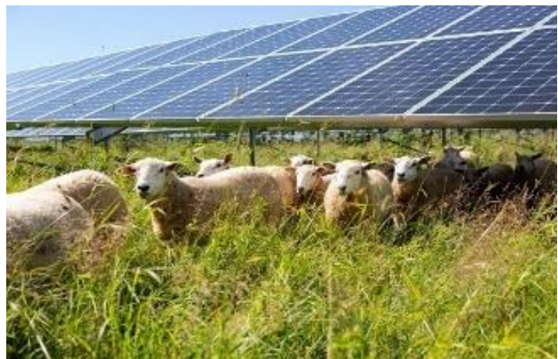
Fig. 5-2. An agrivoltaic system integrating sheep grazing and solar electricity production on farmland
