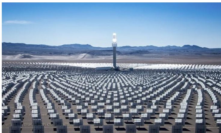
Fig. 3-8. The first utility-scale, 110 MW concentrating solar plant Crescent Dunes Solar Tower in Nevada
