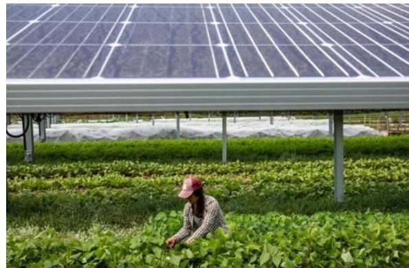
Fig. 5-1. An agrivoltaic system concurrently growing crops and producing solar power on the same farmland
